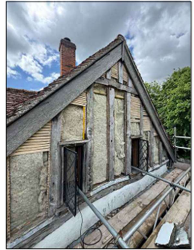
Remove hard cement render from gable. Replace with lime on lath.
