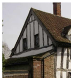
The images left show the north gable above the lean-to roof, the panels removed, and the finished work.
