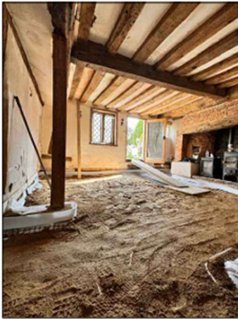
Ceiling timbers and underside of floorboards cleaned using CO2 system
